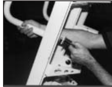
Bolting Handrails to Stair
